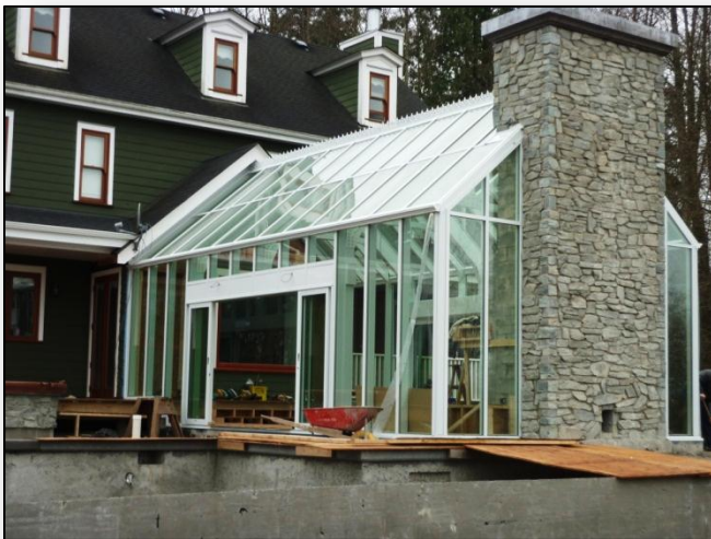
Customization: Fitting around a chimney
